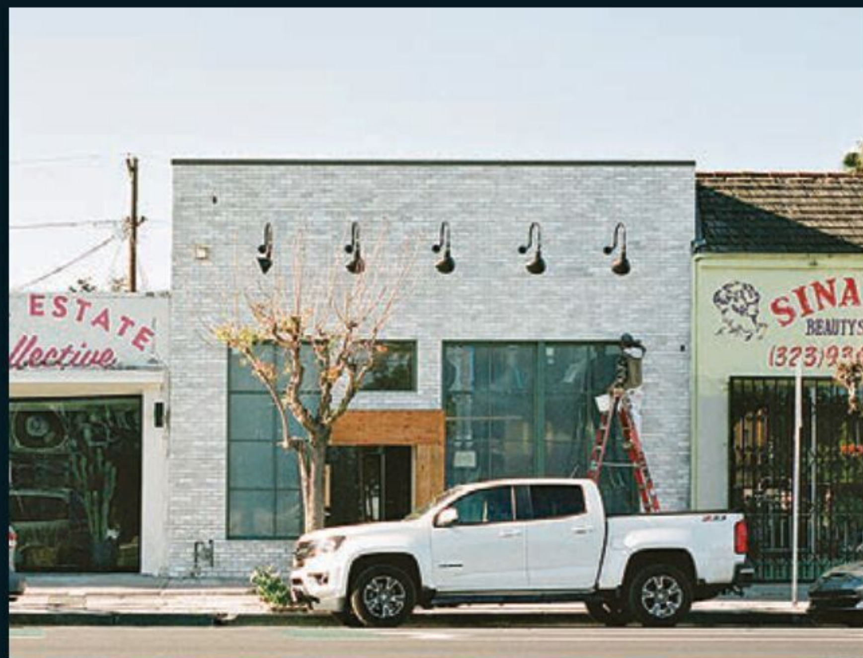
A renovated storefront at 5410
